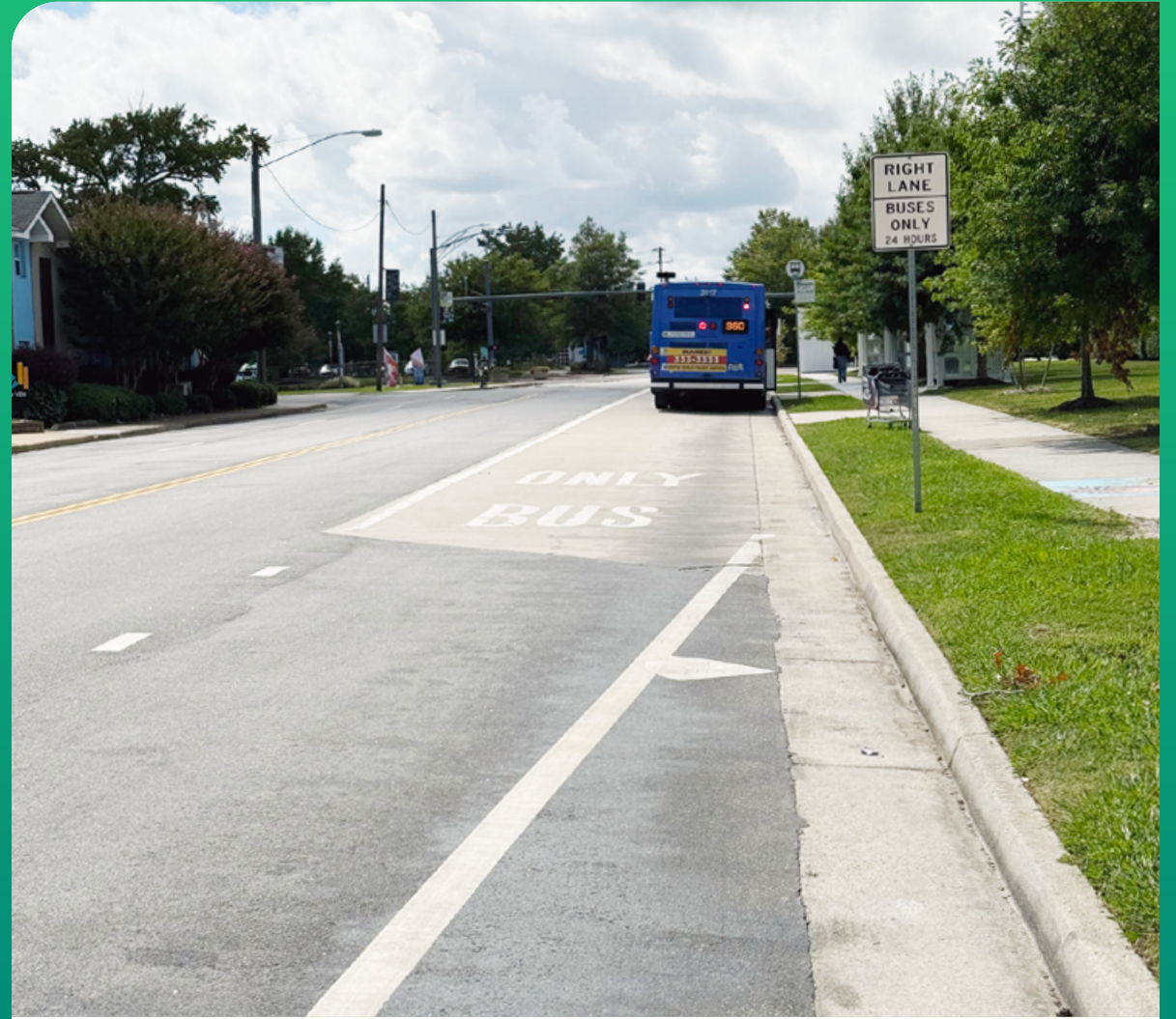
Concrete Pavement at Bus Stop
