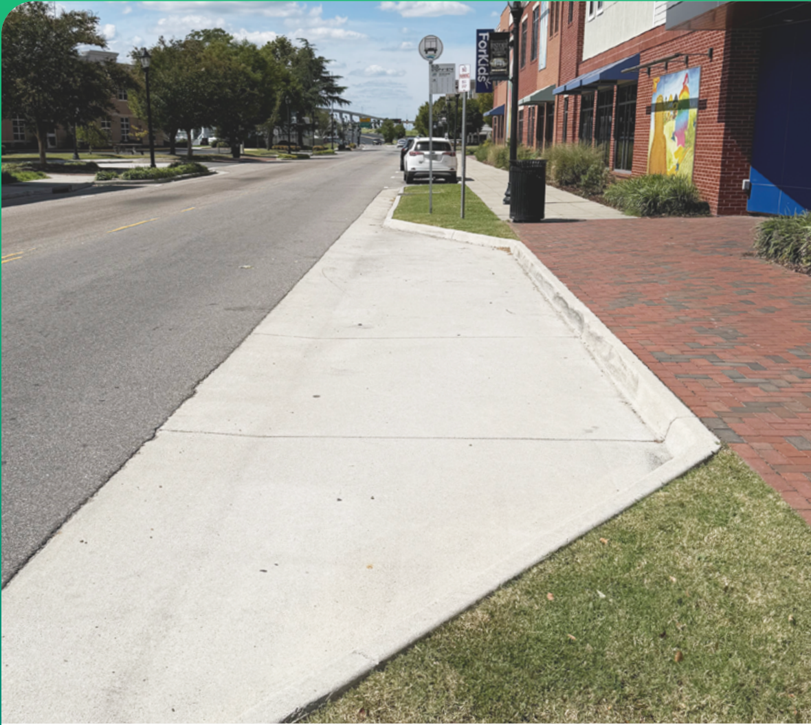
Concrete Turnout at Bus Stop
