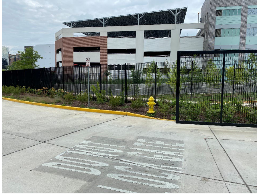
Figure 2 - Added Fire Hydrant in Vicinity of PV Canopy
