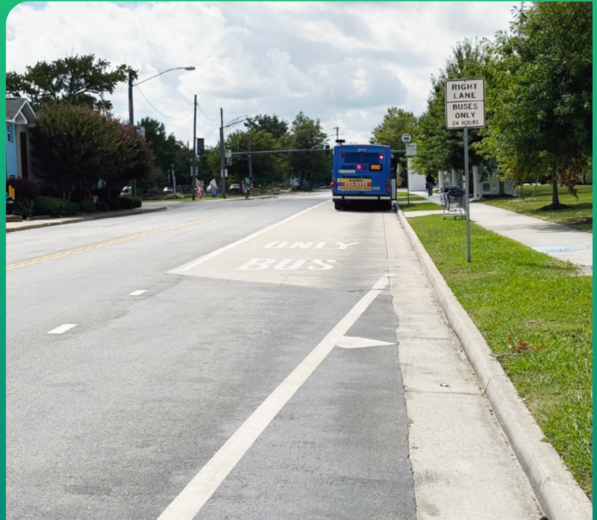
Concrete Pavement at Bus Stop
