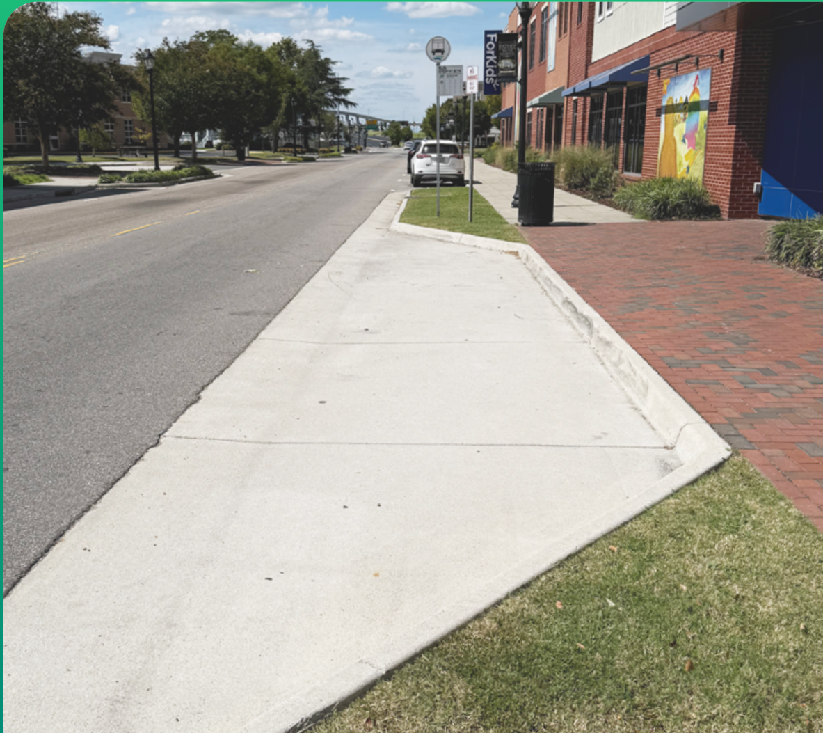
Concrete Turnout at Bus Stop
