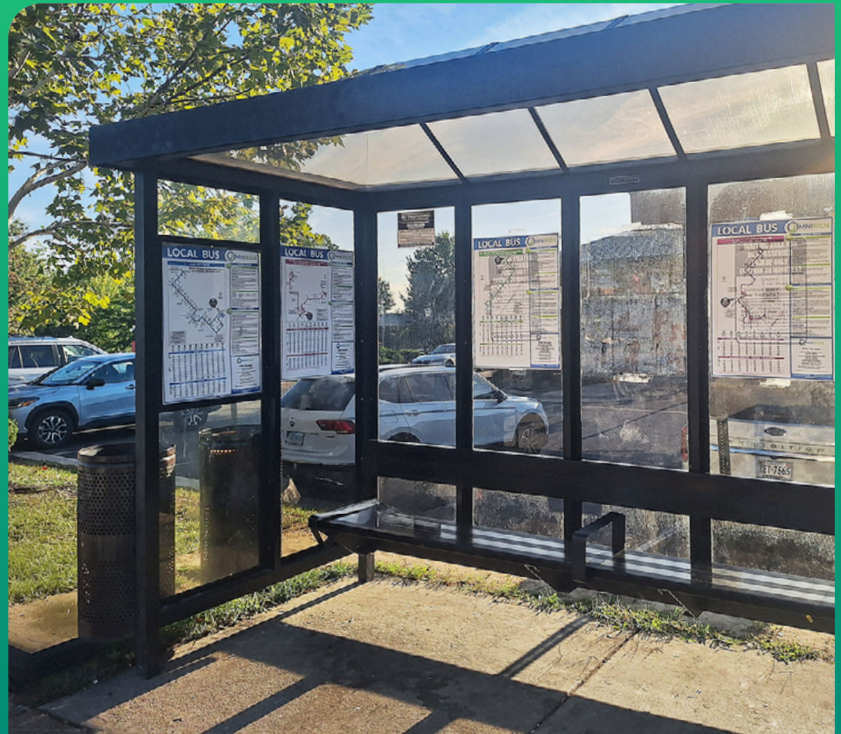
Shelter-Mounted Trash Cans
