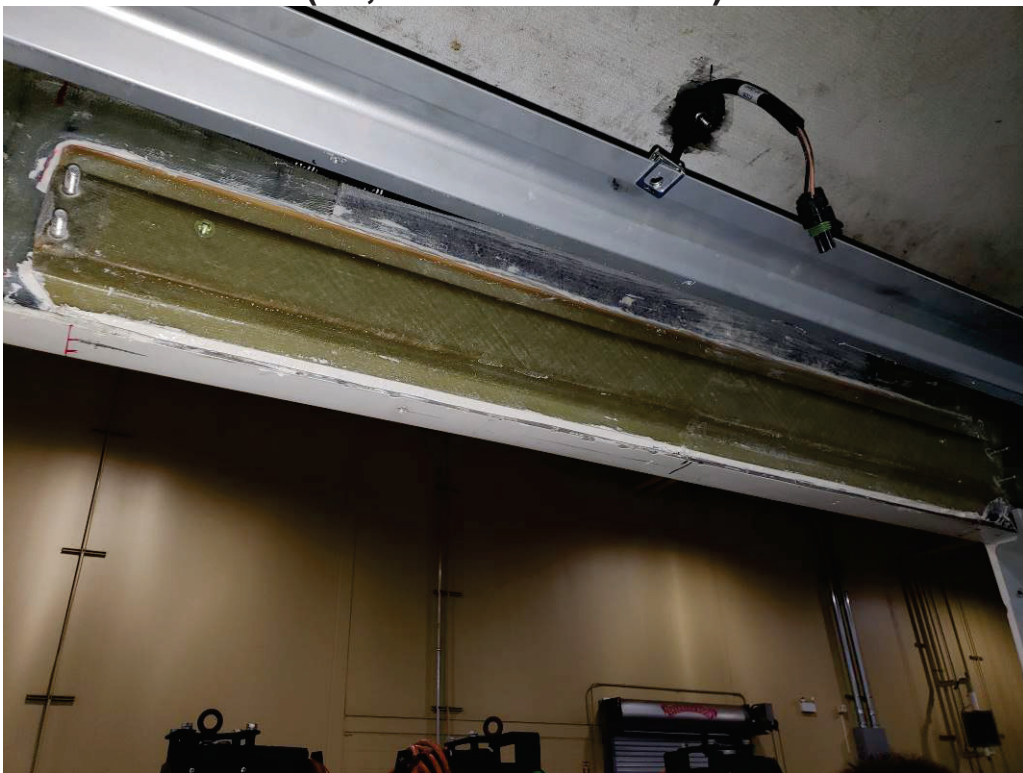
REAR DOOR HAT BRACKET REPAIR (12,999 TEST MILES)
