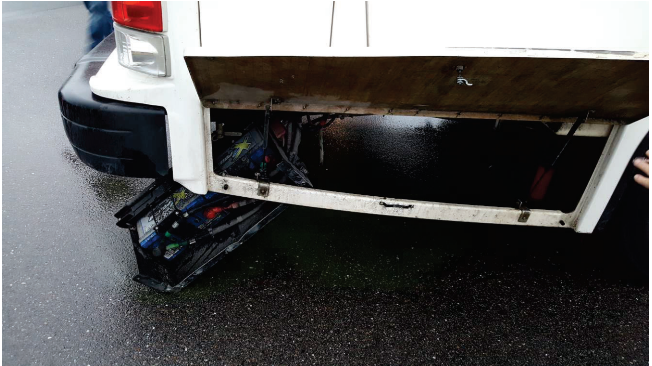
24 VOLT BATTERY BOX FELL OUT (9,334 TEST MILES)
