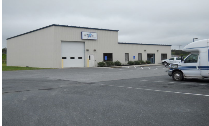
Transit Facility in Tasley
