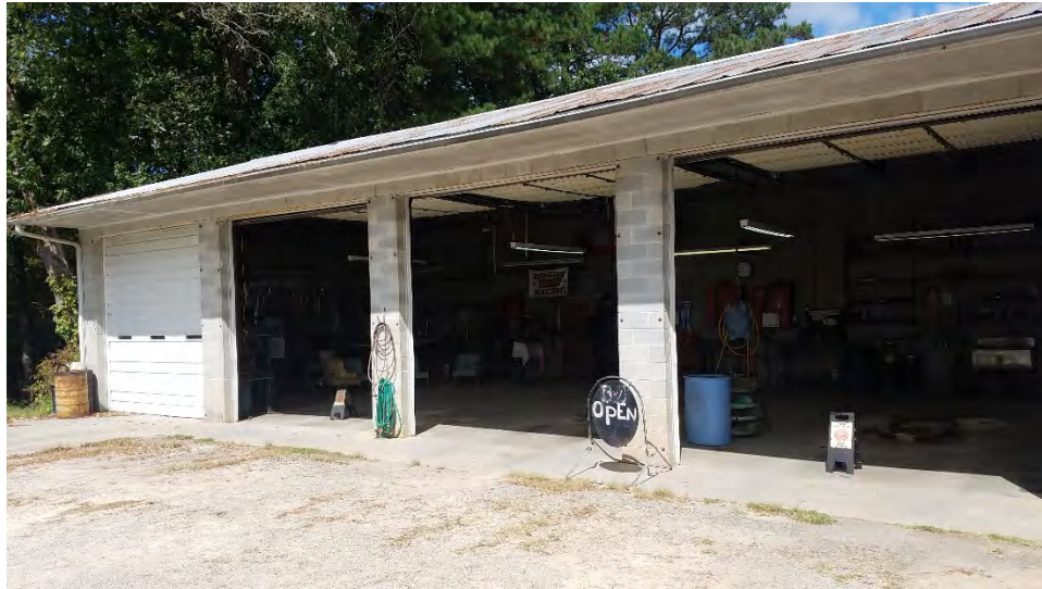
Figure 2-7: LAB South Hill Maintenance Facility
