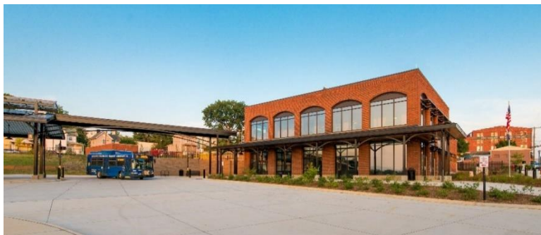
Figure 17: GLTC Transfer Station
