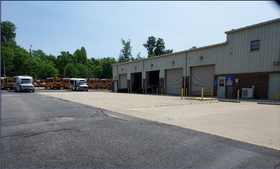
Figure 1-6: City of Danville Administrative and Maintenance Facility
