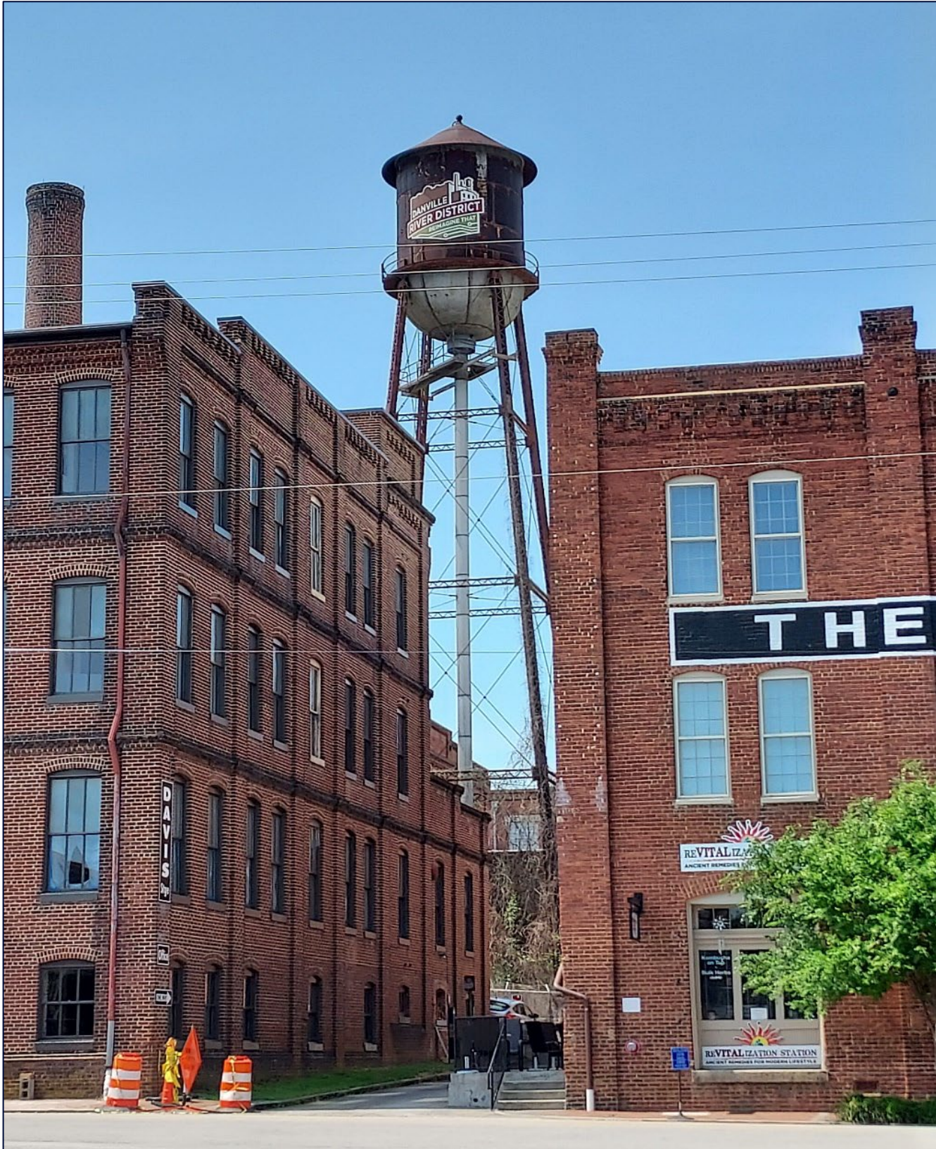
Figure 1-3: Danville River District Buildings Under Renovation
