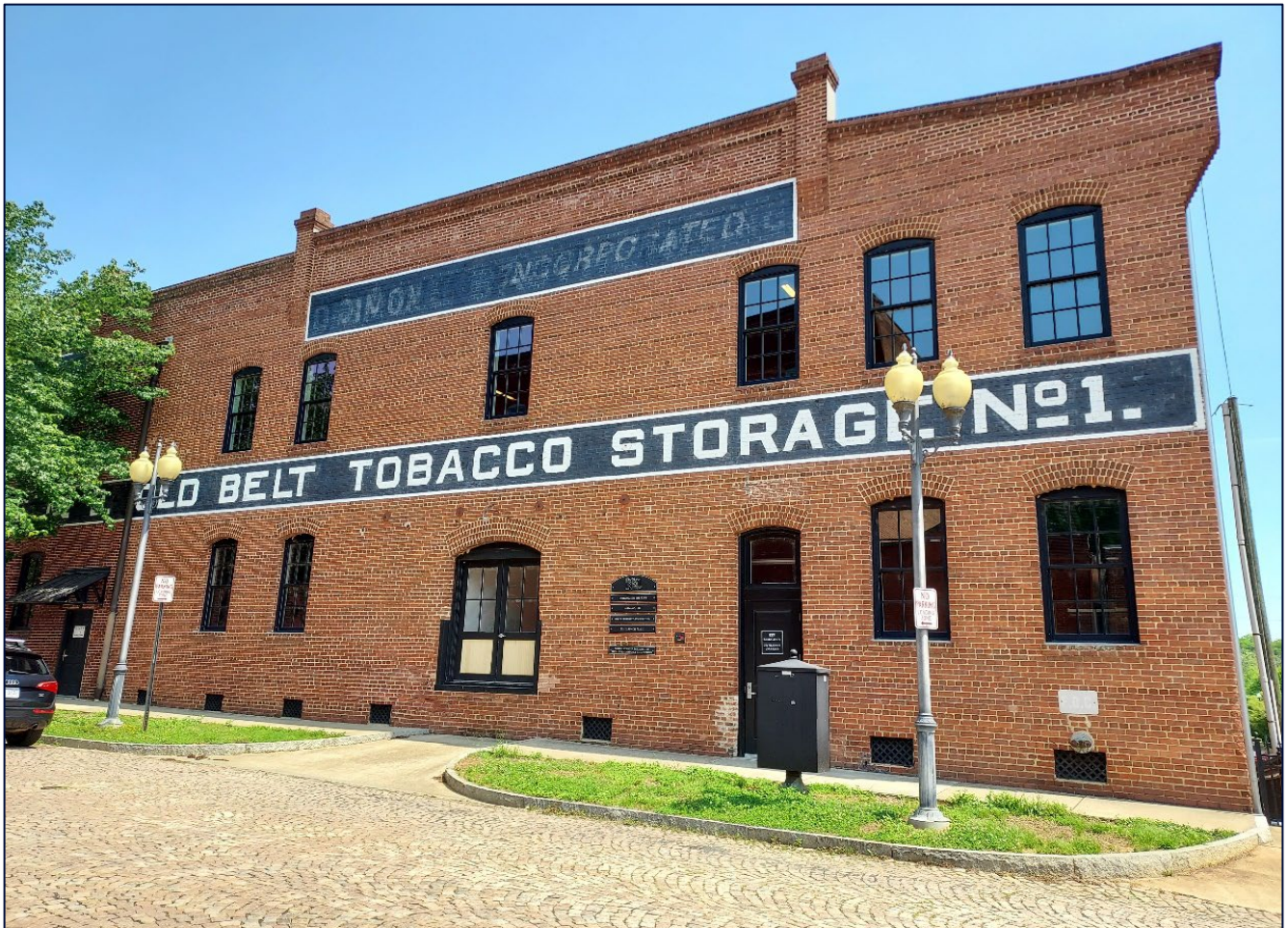
Figure 1-2: Old Belt Tobacco Storage Building
