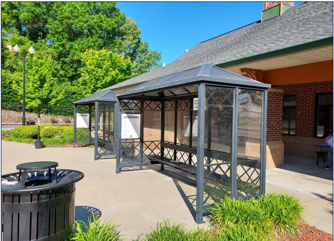
Figure 1-8: Danville Transit Bus Shelters at the HUB
