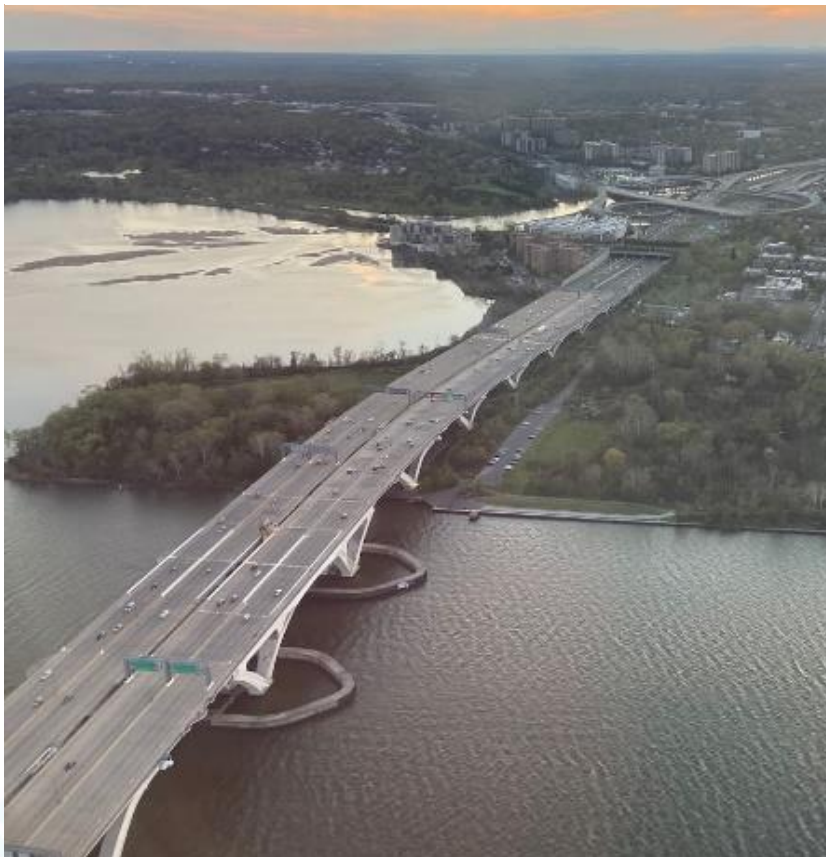
Figure 3. Woodrow Wilson Bridge
